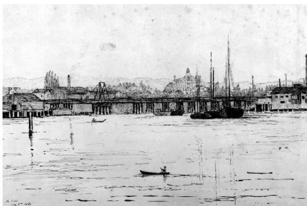
Rock Bay Bridge (1895) 31
