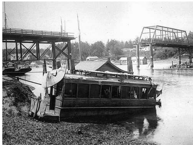
Aftermath of the Point Ellice bridge disaster 29
